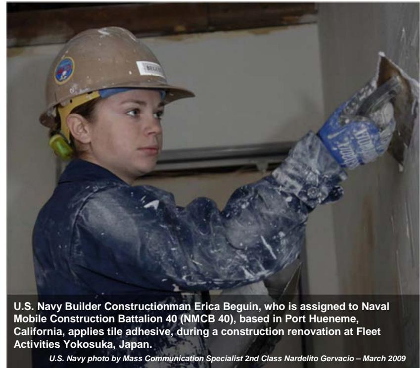
U.S. Navy Builder Constructionman Erica Beguin, who is assigned to Naval Mobile Construction Battalion 40 (NMCB 40), based in Port Hueneme, California, applies tile adhesive, during a construction renovation at Fleet Activities Yokosuka, Japan.
